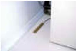
Locate the water/leak sensor on the floor beneath the supply hoses
