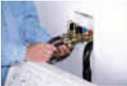
Connect the water supply hoses to the FloodStop valves.
