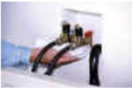
Turn on manual valves (hose bibs) and check for any leak.
