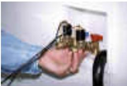
Attach/screw the FloodStop valves onto the manual valves (hose bibs).
