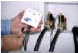
Connect 6-pin connector to the FloodStop control unit.
